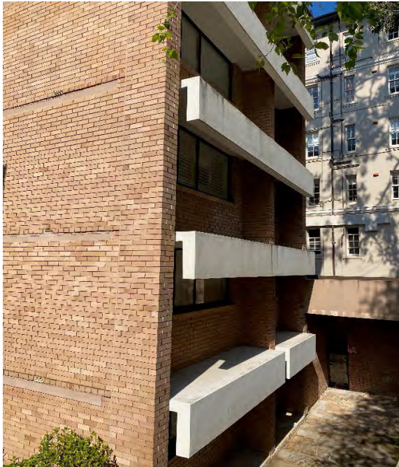
Figure 4.4 The concrete spandrels are expressed on the main elevations.
