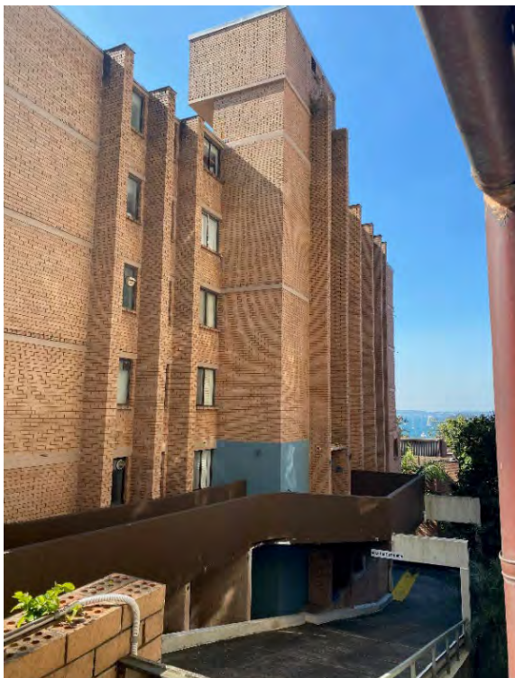
Figure 4.6 Ramped vehicular entry at Onslow Avenue, and the side elevation of brick fins and lift tower.
